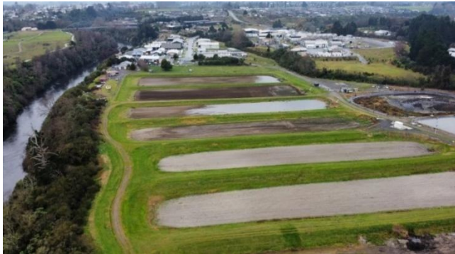
Figure 2 - Rapid Infiltration Beds in the forefront.
